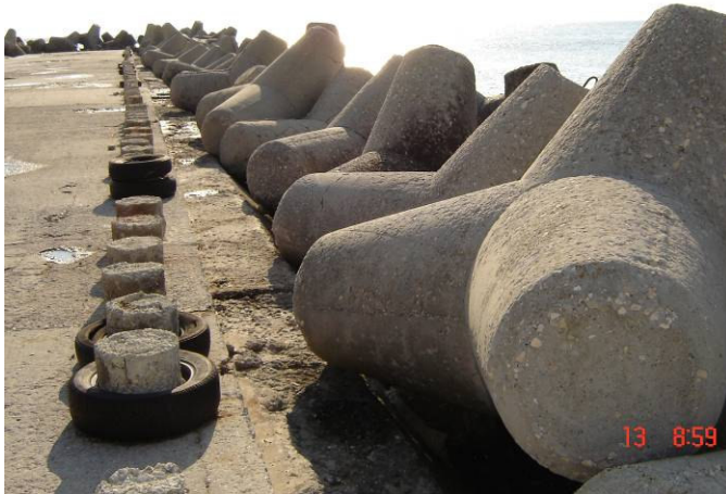
Fig. 4.3 Seaward direction breakwater St. Constantine, with Tetrapods on the right side of the breakwater
