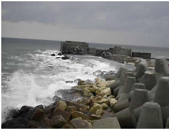
Fig. 2.9 Breakwater made of concrete blocks, natural rocks, and Tetrapods.
