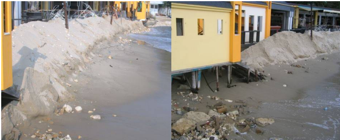
Fig. 1.1 A bar at the Varna beach, that is taking direct damage by wave attack every day.
