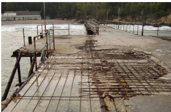
Fig. 2.7 Jetty 2, damage of construction.
