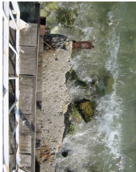
Figure 4-22 Old connection of boardwalk with the collapsed jetty
