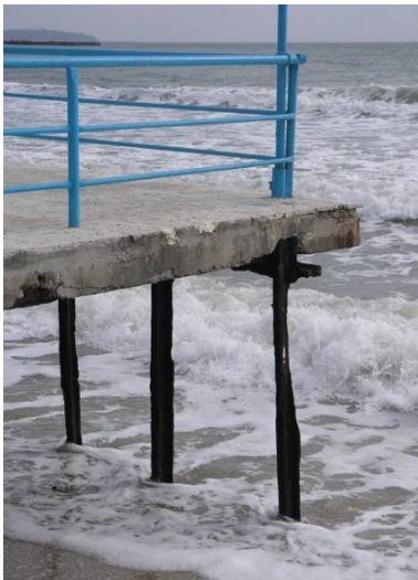
Figure 4-10 Damaged balcony and substructure in 2005
