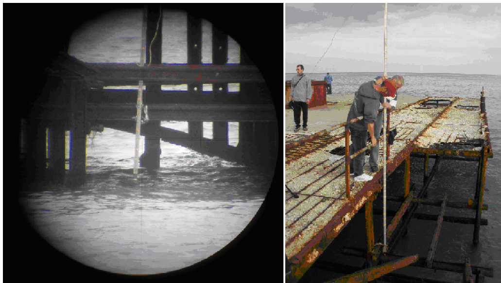
Figure 2-1 Left side the pole and the attached measuring rod, right side installation of the pressure meter and measuring rod
