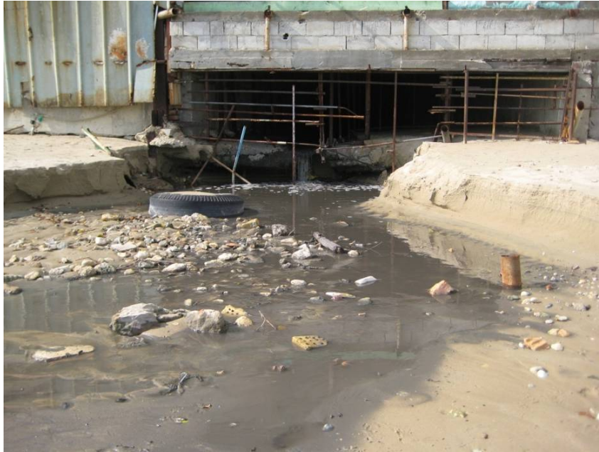
Figure 4-18 Damage to beach by discharge of drainage system.
