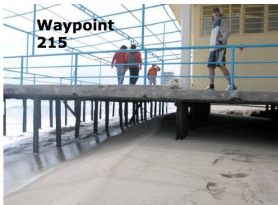
Figure 4-8 Balcony in 2005. Two rows of columns beyond the last wall of the building.
