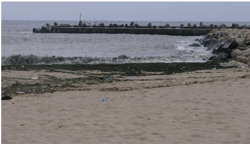
Figure 4-5 Accretion on northside of the Y-groyne 2005
