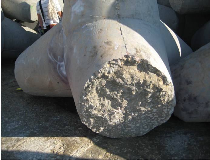
Figure 20 Broken tetrapod
