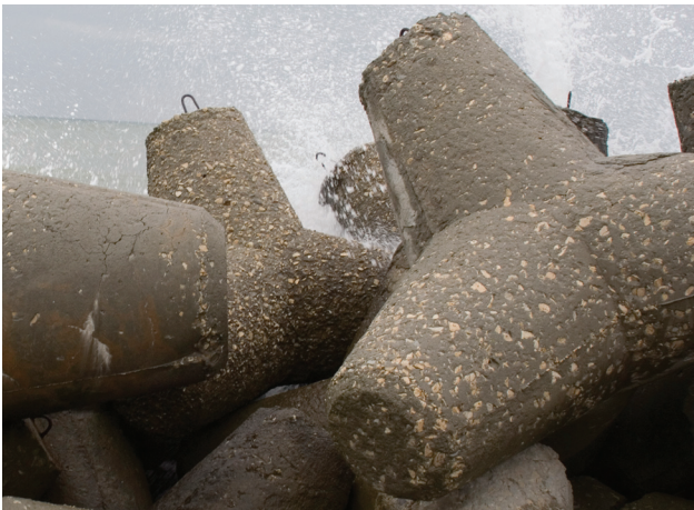
figure 7.1 Concret grains visible
