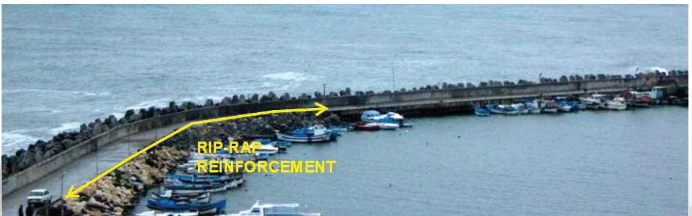
figure 7.5 Rip rap reinforcement
