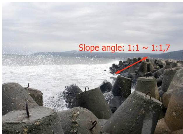
figure 7.6 Slope angle of tetrapods
