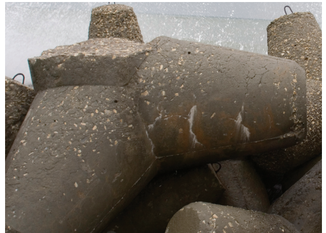
figure 7.2 Broken tetrapod
