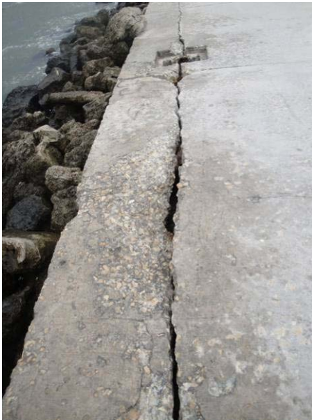
Figure 30: At some points the size of the crack reaches a width of 5 cm.
