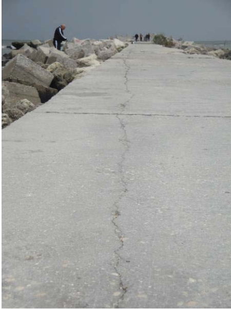
Figure 29: Overview of the crack following the length of the breakwater.
