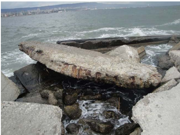
Figure 37: A large piece of the surface plate is broken.
