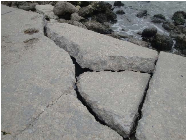
Figure 36: Large cracks in the surfaces plates.
