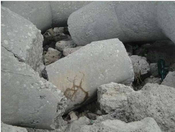
Figure 33: Broken leg of a tetrapod.
