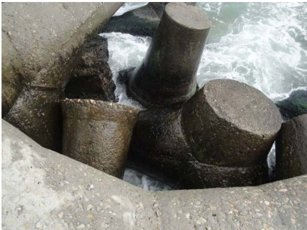
Figure 34: Broken leg of a tetrapod, at construction line.
