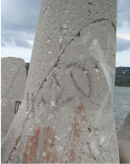
Figure 32: Result of poor construction, construction line clearly visible in tetrapod.
