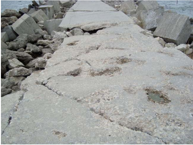
Figure 35: Totally destroyed surface plates.
