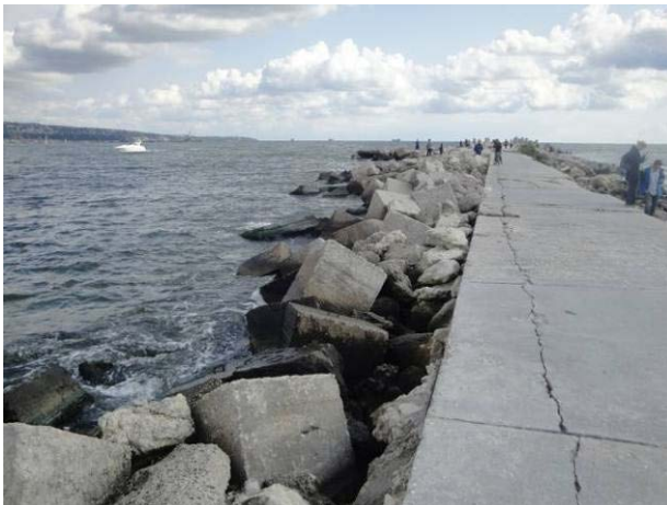
Figure 26: Mixture of concrete blocks and natural rocks.
