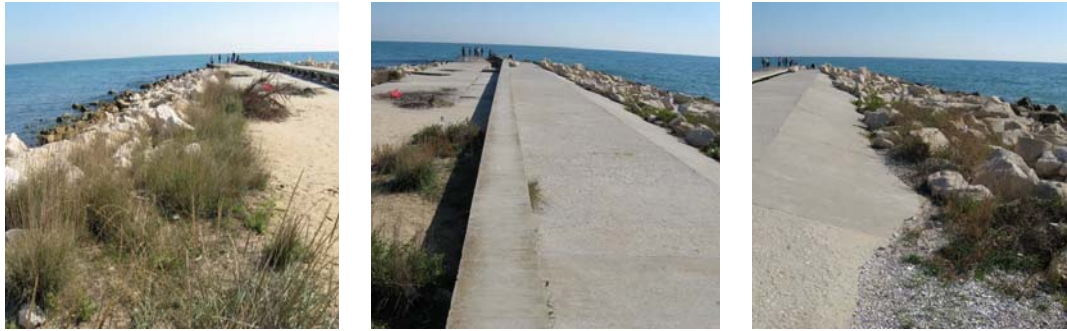
Figure 3-2: Armour rock North-side (left), Caisson core (middle), Armour rock South-side (right)
