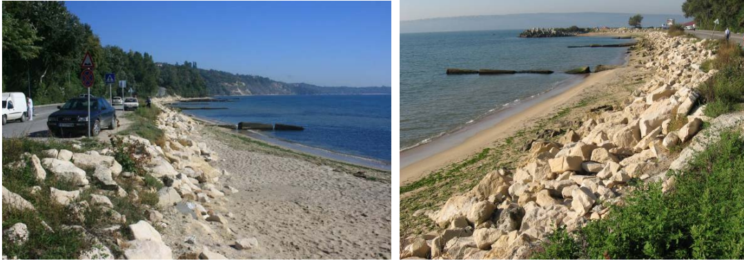
Figure 7-5: Beach east of small groyne, stone revetment and collapsed groynes. Left: view from small groyne towards the east. Right: view on the small groyne from the west.
