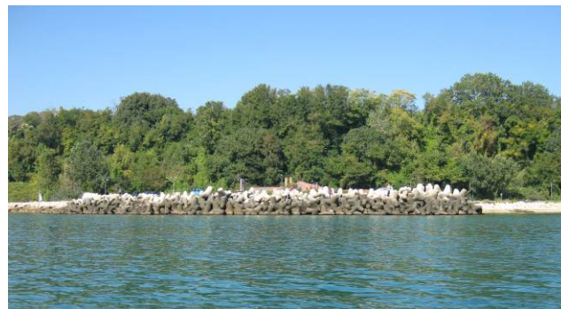
Figure 7-4: Small groyne with Tetrapods as seen from the water
