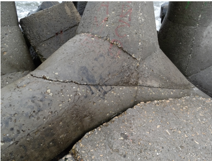
Figure 3-27 Broken tetrapod
