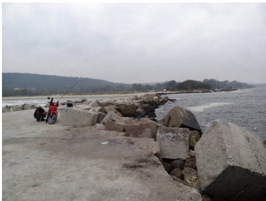
Figure 3-19 Randomly placed cubes
