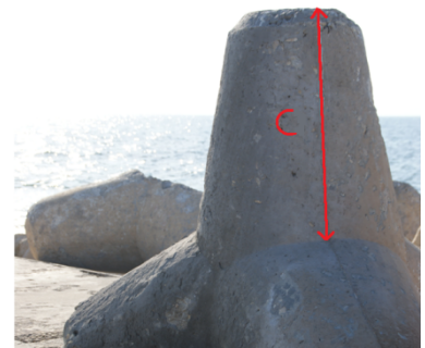
Figure 3-28 Leg length of tetrapod
