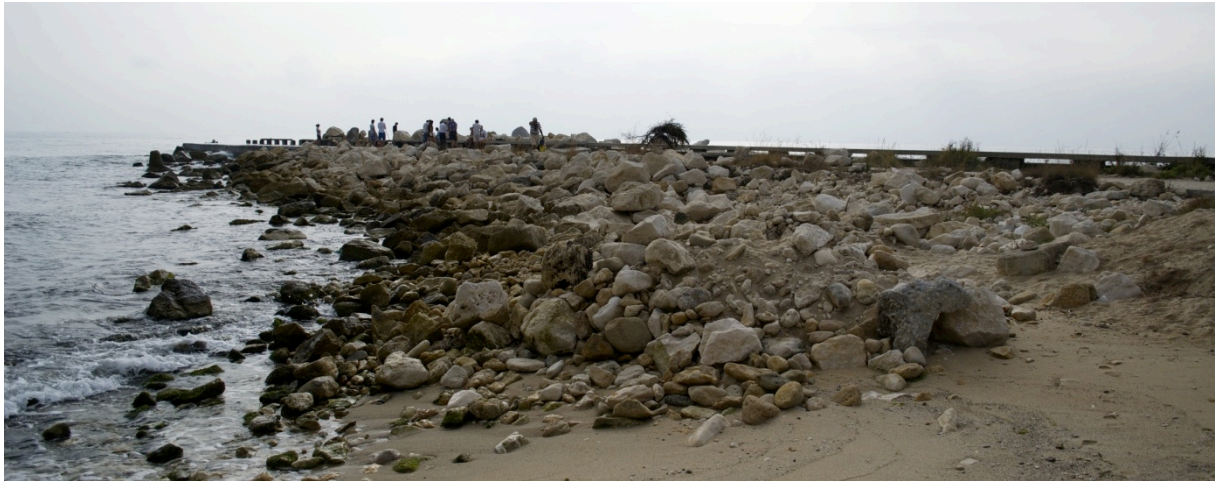
Figure 5-10 North side of the groin (almost no tetrapods are visible)
