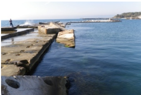
Figure 5-23 Overtopping and washed away elements
