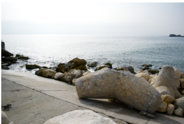
Figure 5-5 Broken tetrapod
