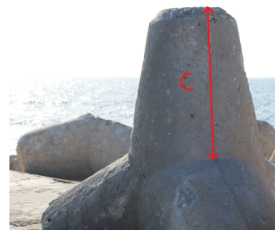
Figure 5-3 Leg length of tetrapod
