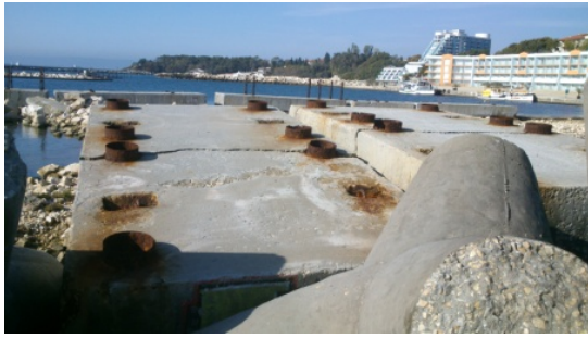
Figure 5-21 Eroded elements
