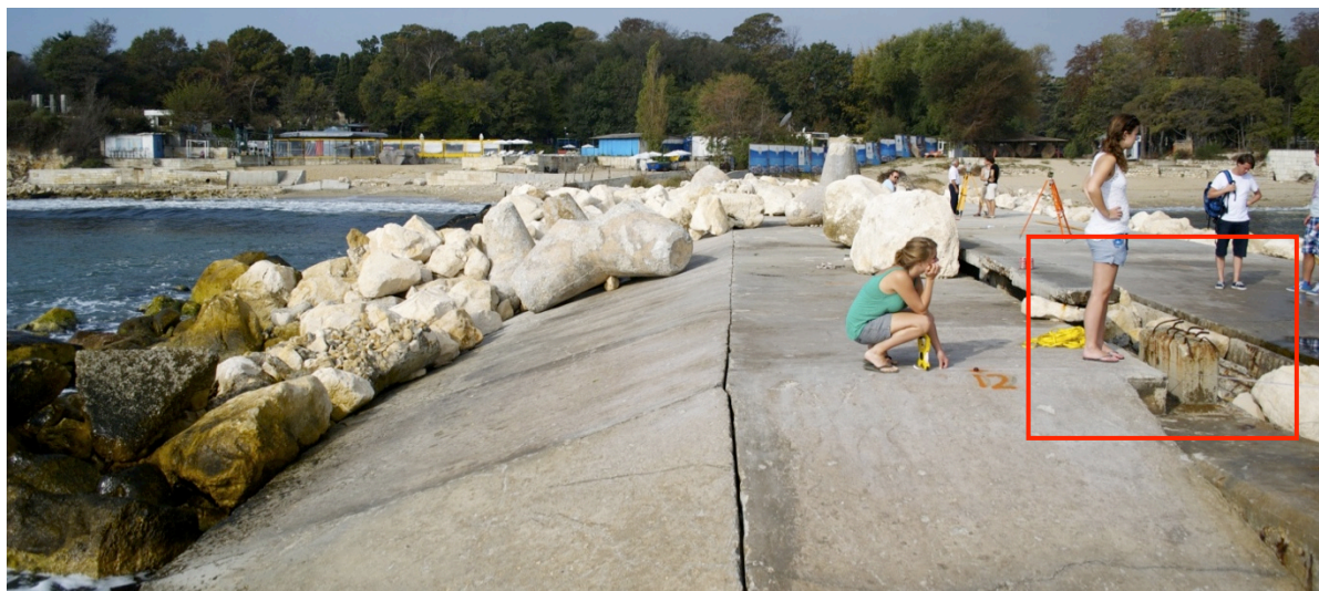
Figure 5-7 South side of the groin (several (broken) tetrapods are visible)
