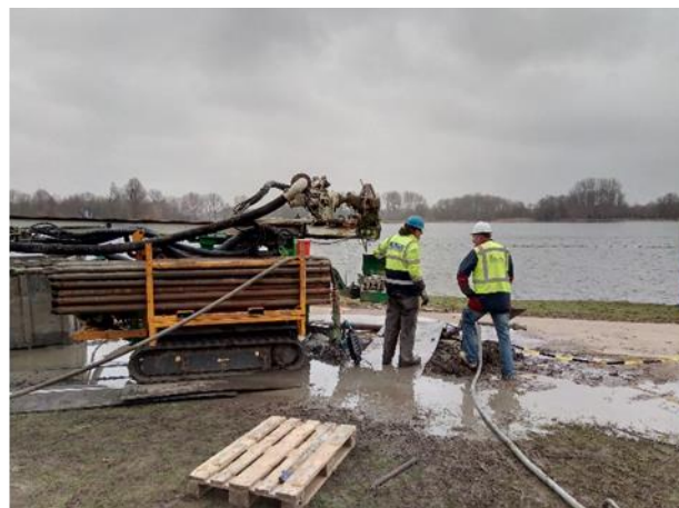
Drilling of DAPGEO-02-01B (50m)
