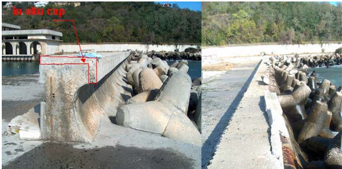
Figure 2.6: Left: Parapet-structure with cap and Tetra pods in front Right: Broken in-situ concrete cap
