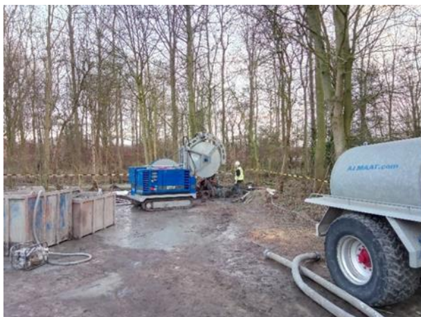
Grouting of DAPGEO-02 (200m)
